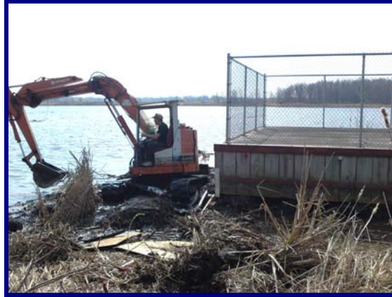
Excavation of overgrowth around Lake Ellen weir structure April 2010
