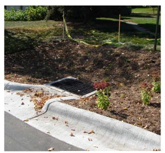
The City of Lindstrom partnered with the Chisago Soil & Water Conservation District to solve erosion problems that were occurring at the end of Linden Street, a dead-end road with a steep slope to the lake. This project has two curb cut rain gardens at the top of the hill, on either side of Linden Street. These
